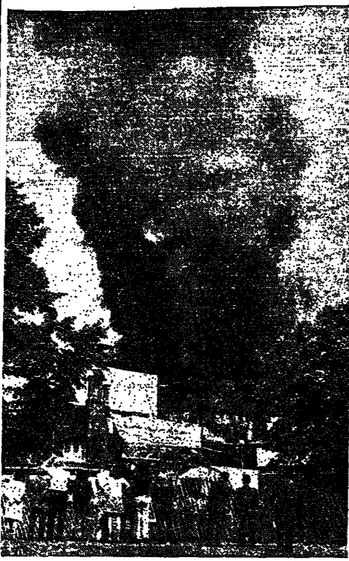
Fire yesterday partly destroyed a £4m beer fermentation plant being built for Watney Mann at Mortlake, Surrey.
